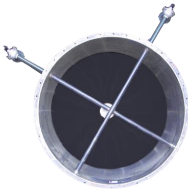
Auto-Booster / Duct Cleaner in 64 inch Duct
