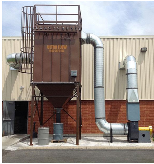
V-Series top bag removal for larger dust collection
