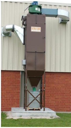
LC-Series bottom bag removal
